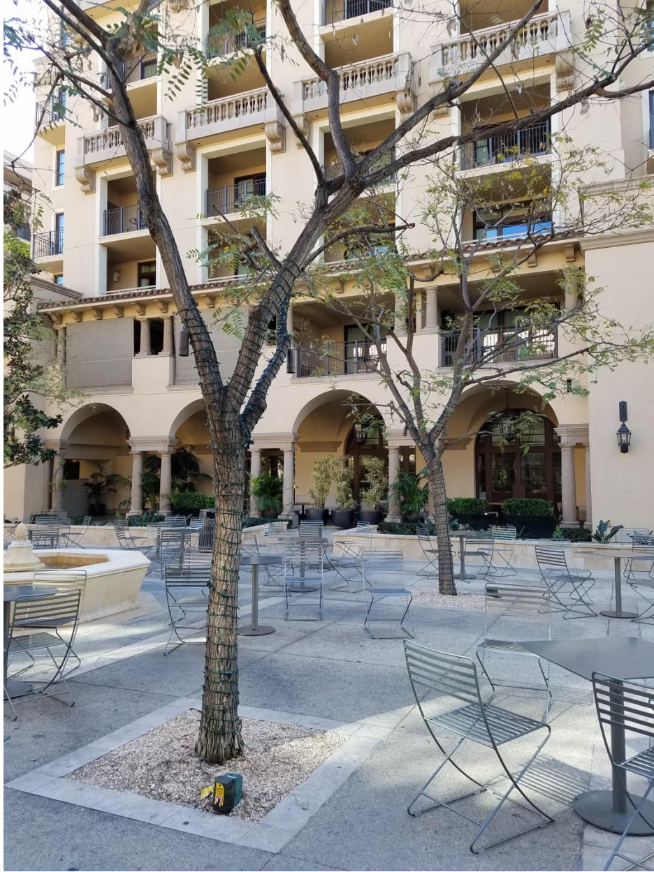
Example of Decorative Tree LED Lighting Beverly Canon Garden
