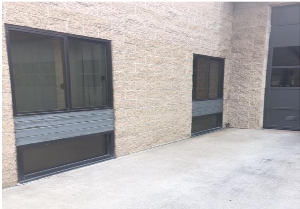
Photograph 2: View of lead containing brown exterior window frames.
