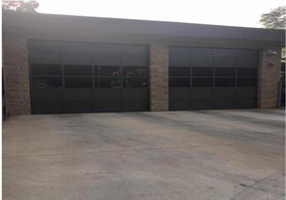
Photograph 1: View of Fire Station #2.
