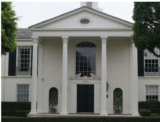
9370 Santa Monica Blvd., close-up of the front (north) façade. Note the pedimented entrance portico with Corinthian columns, classical door surround, and arched niches (ARG, 2019).
