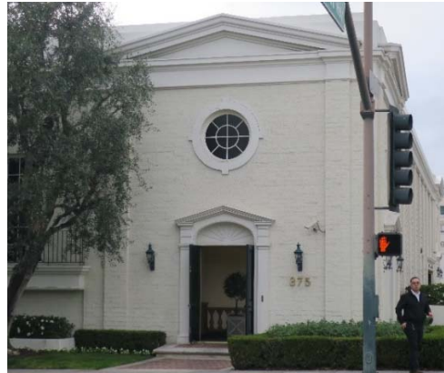
375 N. Crescent Dr., close-up of the pedestrian entrance at the northeast corner. Note the pediment and entablature at the parapet, circular window, and classical door surround (ARG, 2019).
