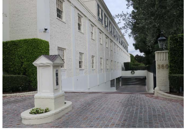
360 N. Crescent Dr., view north of the south facade and parking ramp (ARG, 2019).
