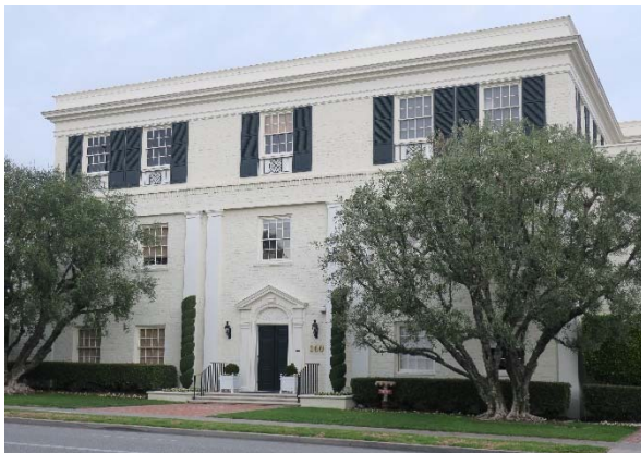
360 N. Crescent Dr., view northeast of the west facade (ARG, 2019).
