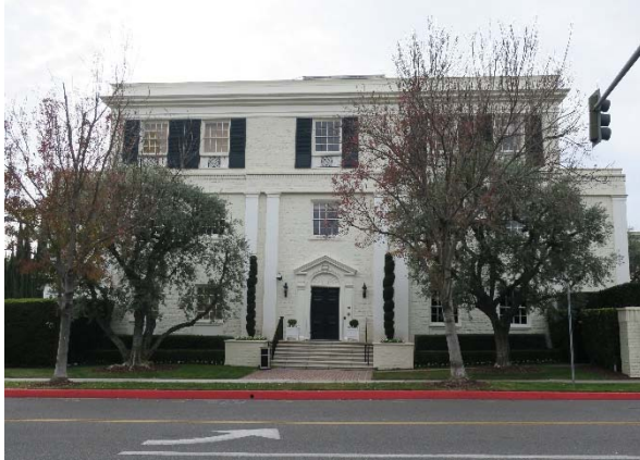
360 N. Crescent Dr., view southwest of the east facade (ARG, 2019).
