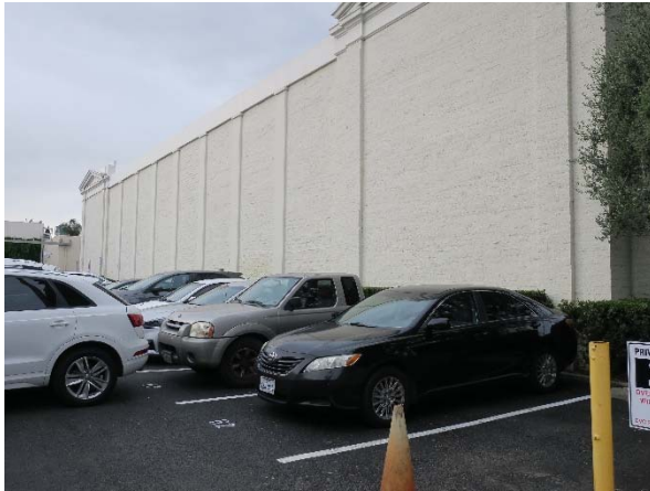
375 N. Crescent Dr., view northwest of the south façade (ARG, 2019).
