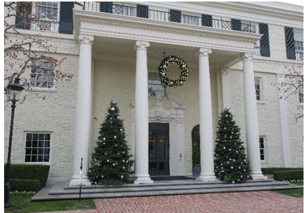
360 N. Crescent Dr., close-up of the front facade entrance portico. Note the Ionic columns and classical door surround (ARG, 2019).
