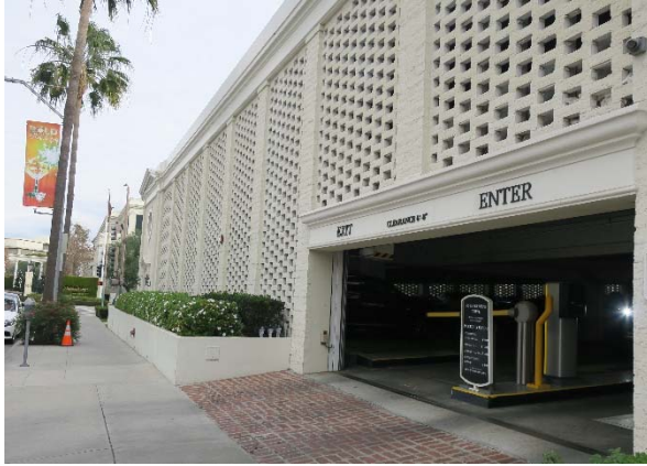
375 N. Crescent Dr., close-up of the vehicular entrance off of Brighton. Note the lintel and cornice above the entrance and wall panels of brick brise soleil (ARG, 2019).
