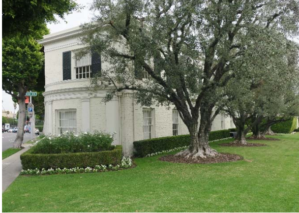
9370 Santa Monica Blvd., close-up of the wing, west end. Note the round bay with pilasters and entablature (ARG, 2019).
