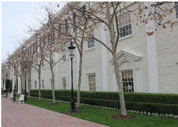
360 N. Crescent Dr., view southeast of the front facade (ARG, 2019).
